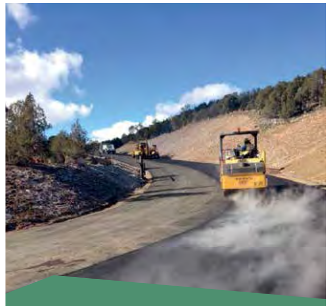
Four Corners Materials, an Oldcastle Materials subsidiary, installed a paved haul road at its Animas Glacier Pit in Colorado, US to reduce dust emissions from the movement of plant and equipment on-site.
