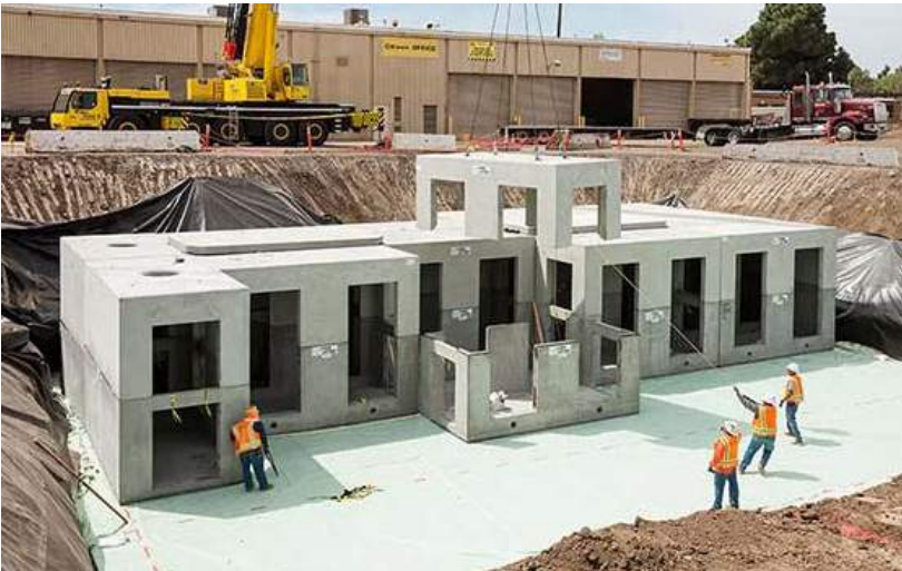
The Metro Expo Light Rail operations and maintenance facility in Santa Monica, California, US, uses Storm-Capture units to harvest and store rainwater for reuse in landscape irrigation and vehicle washing. Oldcastle Stormwater Solutions, part of Oldcastle Precast, was involved in the design and construction of a concrete stormwater management system to reduce the impact on the municipal water supply in this high drought area.
