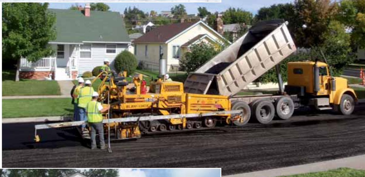
Above: In the US, Oldcastle Materials has pioneered the use of warm mix asphalt (WMA) which requires 15-30% less energy than traditional asphalt. Shown here is the first use of WMA in the state of South Dakota, laid by CRH subsidiary Hills Materials, at a residential neighbourhood in Rapid City. With over 100 WMA plants, CRH/Oldcastle produces circa 5 million tonnes per year.
