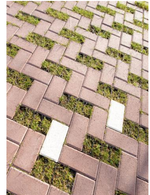
Struyk Verwo Infra, Netherlands, part of our Europe Lightside Division, has developed the Greenbrick concept, which combines paving with grass and makes large surfaces suitable for water infiltration and evaporation.
