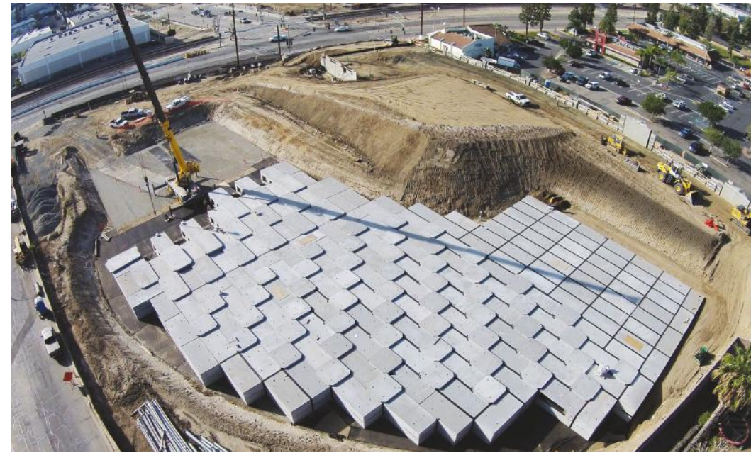
Oldcastle Precast, part of our Americas Products Division, provides a range of solutions for climate adaptation. The Oldcastle Precast StormCapture system, installed at a community development in California, US, captures and treats stormwater, reducing flooding and water quality risks.
