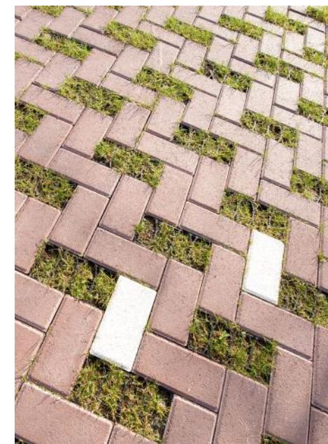
Struyk Verwo Infra, Netherlands, part of our Europe Lightside Division, has developed the Greenbrick concept, which combines paving with grass and makes large surfaces suitable for water infiltration and evaporation.
