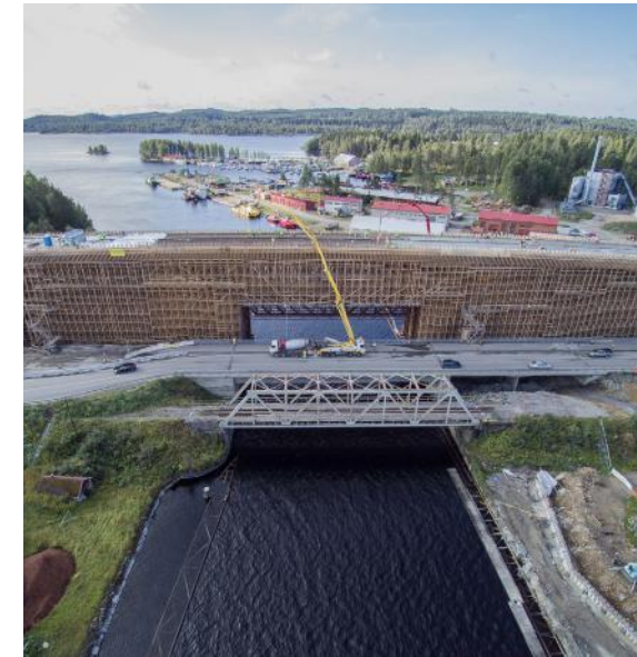
Rudus, a company within our Europe Heavyside Division, delivered 5,000 m 3 concrete to the Laitaatsalmi bridge project, which at 500 metres in length is the longest prestressed concrete bridge in Finland. The concrete was produced using CEM II cement and the maximum amount of blast furnace slag was used as mineral additive.
