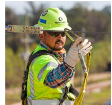
Safe working practices and personal fall protection reduce safety risks of working at heights for workers at Gulf Coast, part of our Americas Materials Division as seen at this Port of Beaumont project in Texas, US
